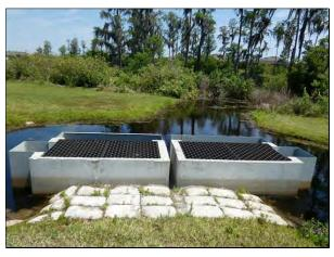
Stormwater Drainage Control Structure
