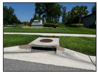
Stormwater Drainage Curb Inlet
