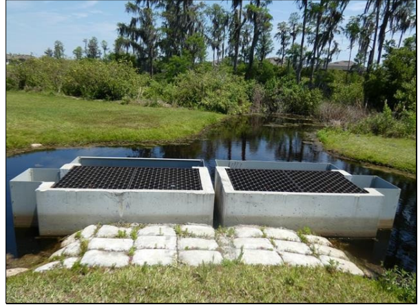
Stormwater Drainage Control Structure
